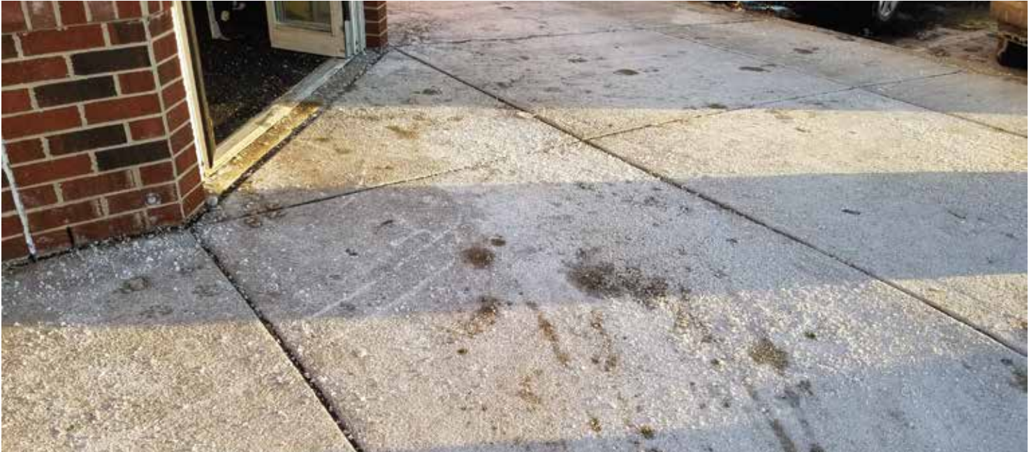
Chloride-based ice melts work well on snow farther from buildings – but the closer they get to entranceways, the more likely their residue will be tracked inside.
