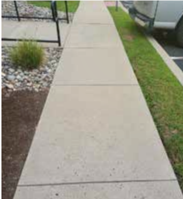
(Sidewalk Before Pre-Treatment)
